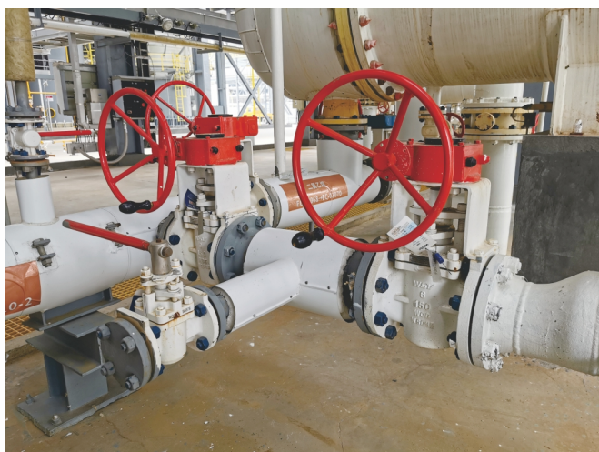
Weidouli sleeved plug valves in Wanhua VCM process line
